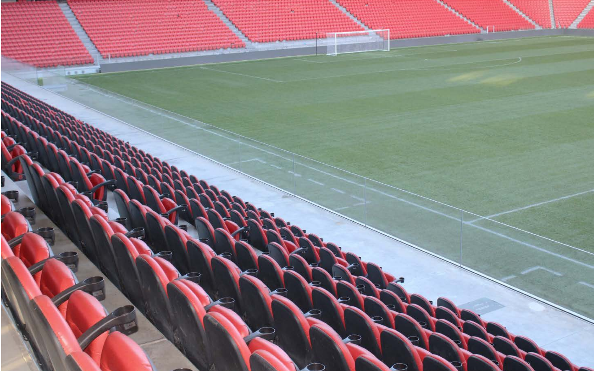
Fig. 18: Interior view of "Air Albania" Stadium
